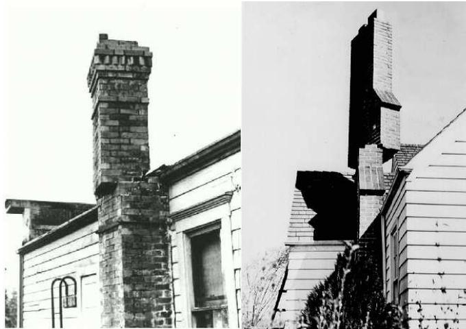
*Figure 2.17: Building damage after a strong earthquake, that may be caused by rotational motion. Left photo is courtesy of the Geological Survey of Canada. Right photo Edwards, 1999.*
