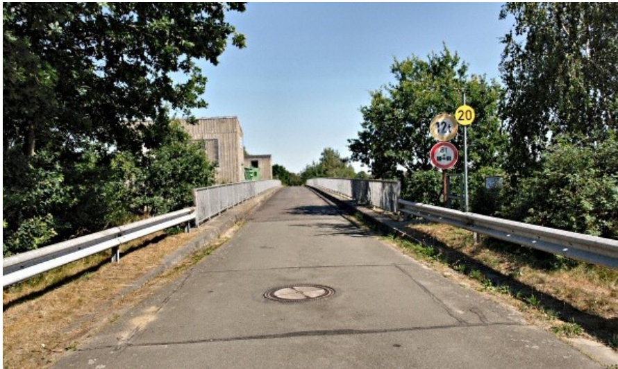
Figure 3.B.1: COVER OF DEMOLITION CHAMBER INSTALLED IN ROAD
