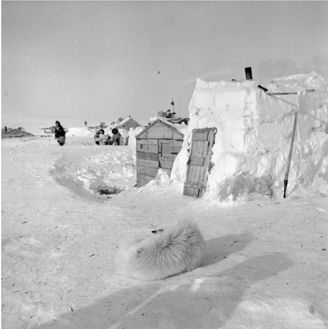
Figure 5. Initial Inuit housing at Resolute Bay. Gary Lunne/National Film Board of Canada. Photothèque/Library and Archives Canada/PA-19142, 1956.
