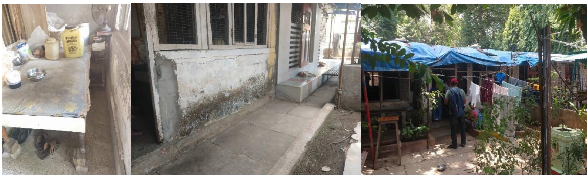
Figure 10 Adaptation efforts at the household level (from left to right): Elevating furniture, raising the house level if affordable, covering the roof with tarpaulin sheets against heavy rainfall, Source: own
