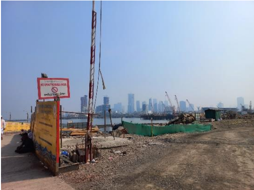
Figure 11 Coastal Road – construction work underway, Source: own
