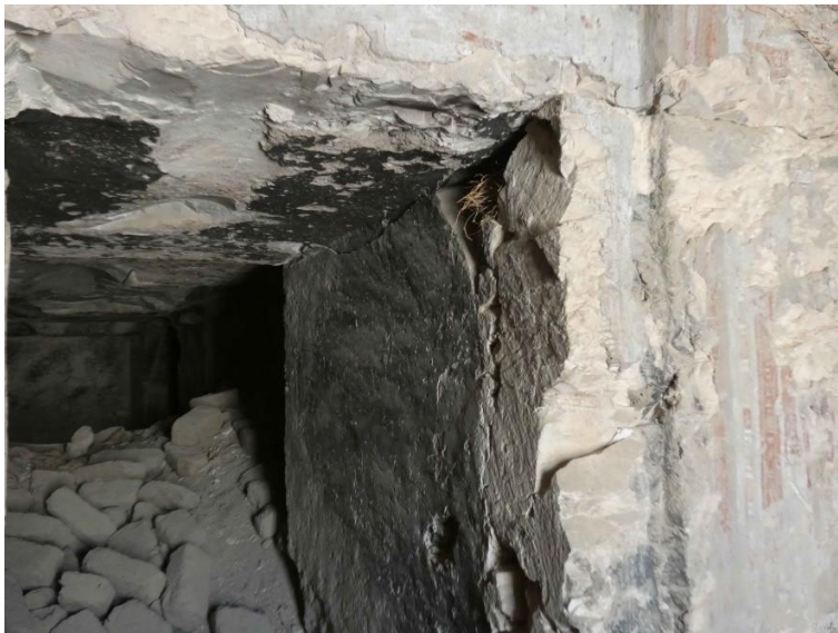
Pl. 91. Southern wall of the passage.
