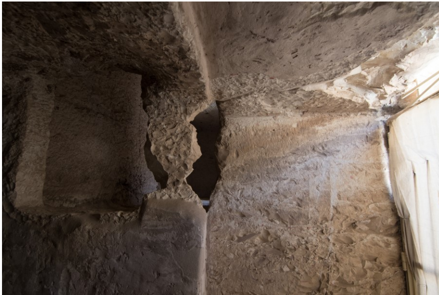
Pl. 120. Breakthrough in the rock-cut wall.
