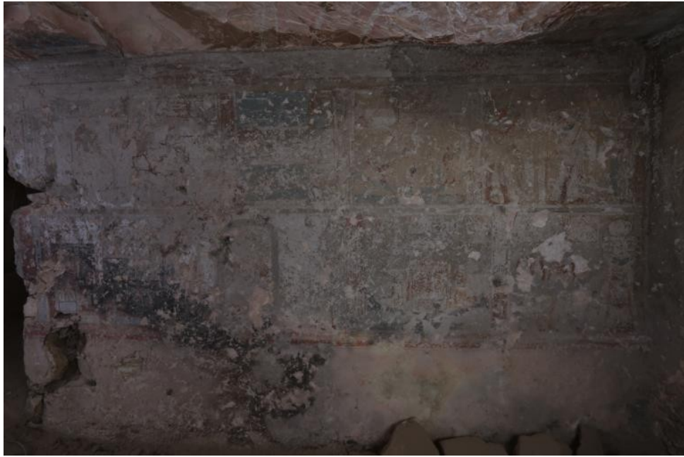
Pl. 92. The west wall northern part of Room 1.
