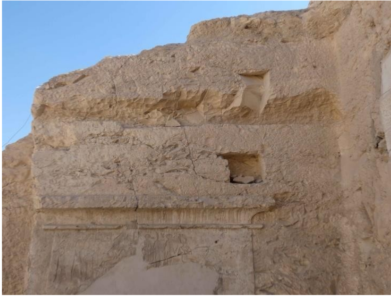
Pl. 44. Emplacement for ceiling slabs.
