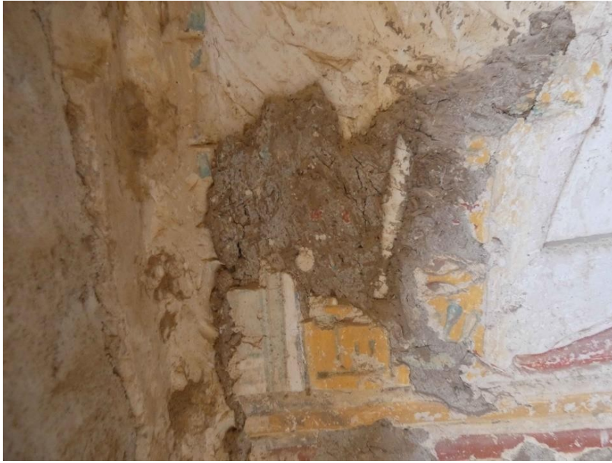
Pl. 80. Ancient reparation of the northern side decoration.
