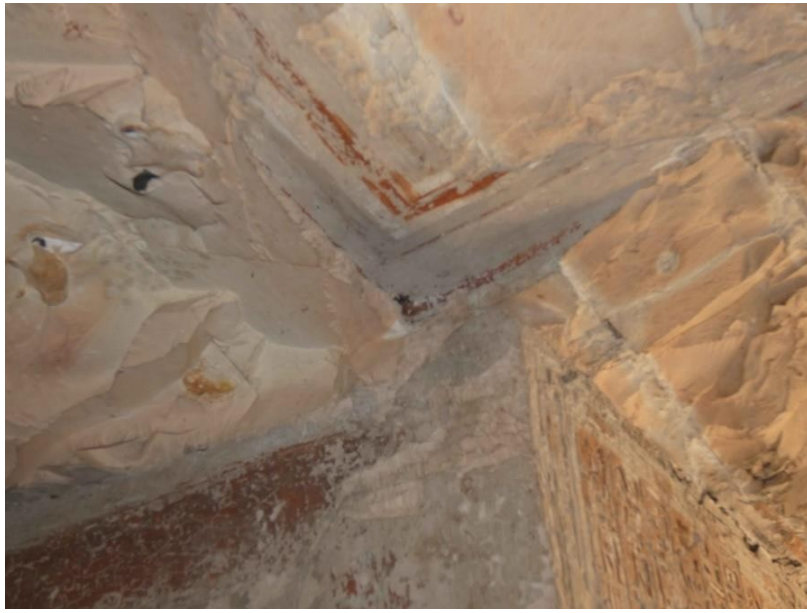
Pl. 83. Smoothing the corner of the ceiling in the western part.
