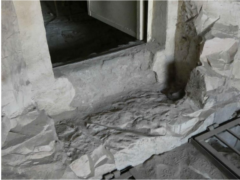
Pl. 29. Lower door socket on the western side of the entrance to the second room.
