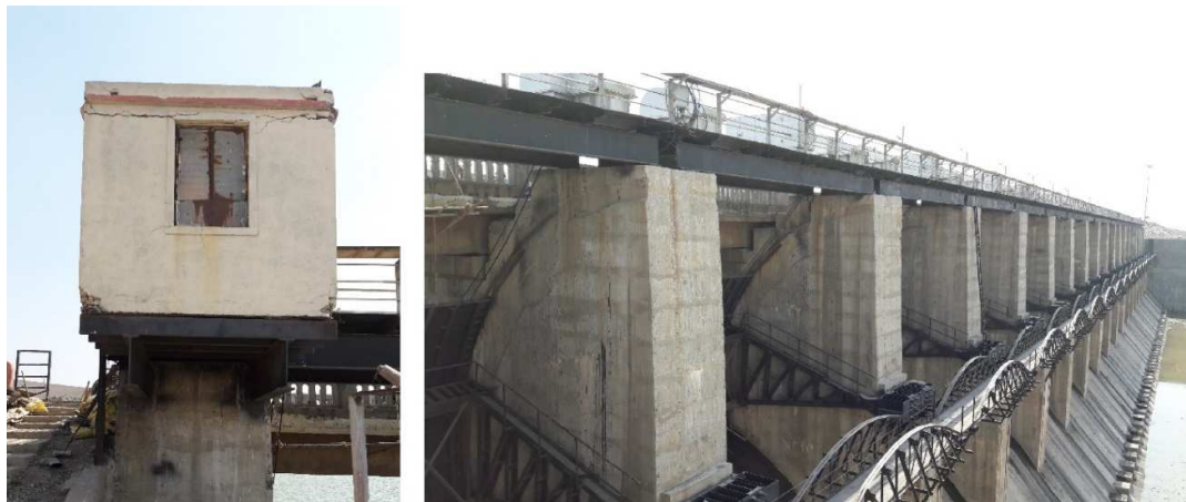
Figure 5.3: Old cabin (left) and concrete spillway (right) on Machhu-II dam. Photo: by author
