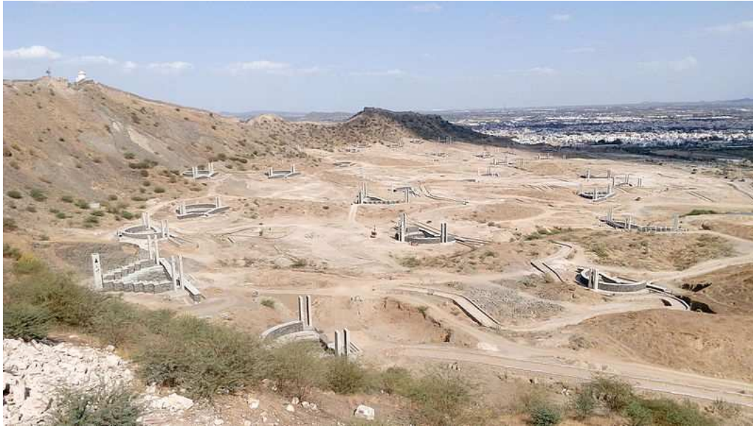
Figure 4.6: SEMM under construction, Photo: Nizil Shah, 2016. Source: https://commons.wikimedia.org/wiki/File:Smritivan_2001_Gujarat_earthquake_memorial_garden_in_Bhuj,_Gujarat,_India.jpg
