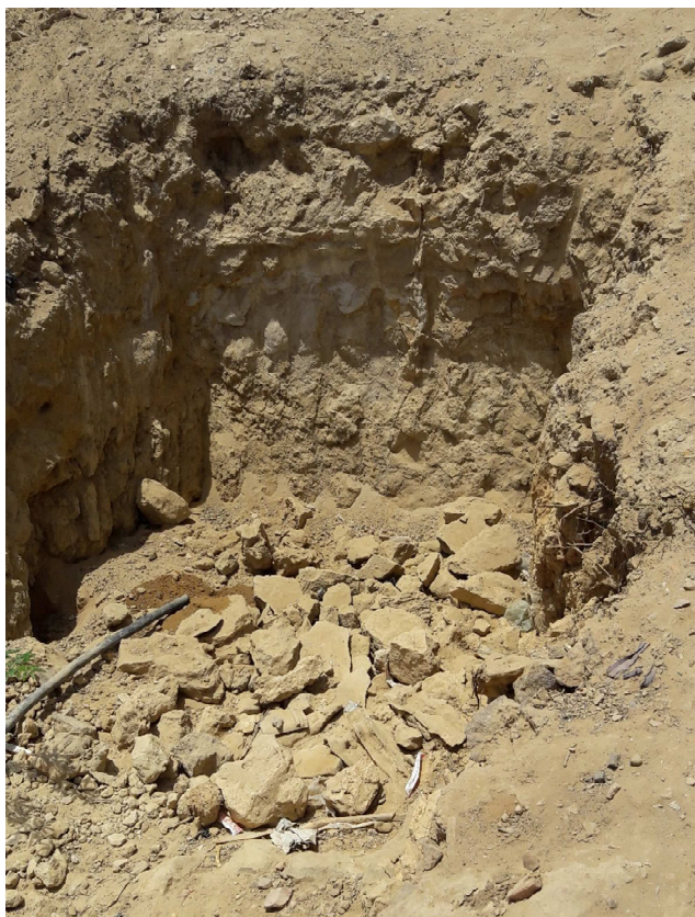
Figure 3.3: Broken water pipe in old Adhoi used by some households for daily needs. Photo: by author
