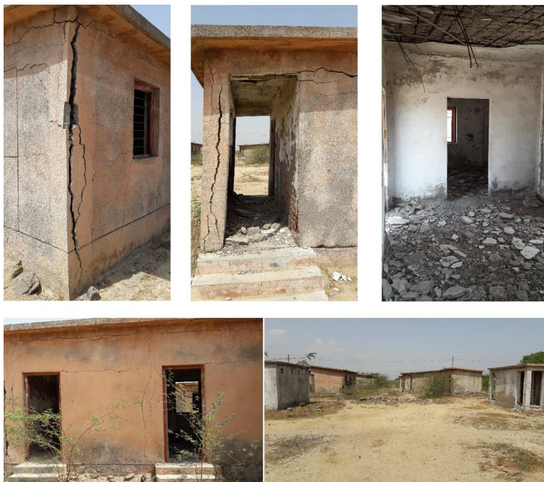
Figure 3.4: Dilapidated condition of houses in New Vondh. Photo: by author
