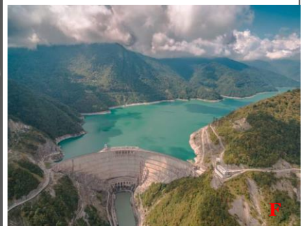
View of the Enguri river dam at the border with modern Abkhazia.
