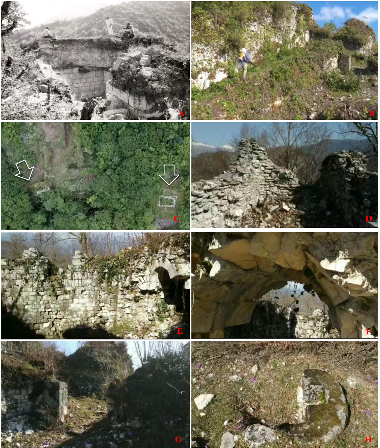
Visualization of structural remains of Tzibile fort and related church. A- View of the Tzibile fort during the excavations in 1970. B- The south-eastern walls of Tzibile fort covered by wood, during the cleaning activities in 2019. It leads up to a massive square tower built in the early 6 th century. C- View of structural components inside fortified area. D- survived part of church. E-F Engineering aspect of construction and part of arched tower. G- Entrance. H- Baptisterium.
