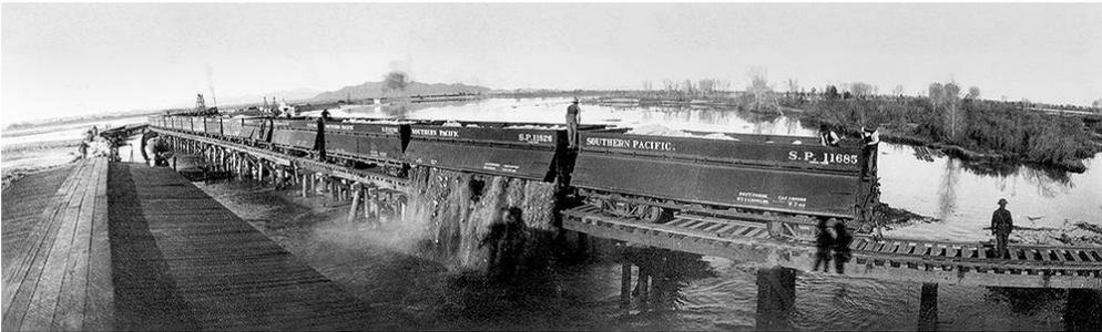
**FIGURE 1.6.** Dumping rock to close the breach, 1906. (Photograph courtesy of the Imperial Irrigation District, "The Great Flood," Greetings from the Salton Sea, <http://www.greetingsfromsaltonsea.com/flood.html>.)
