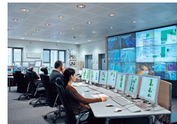
Figure 3.2: Highway Operator Room ©Siemens 12
