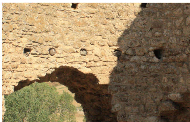
Figure 3.189 : Wooden beams in the inner façade, image by author (2011).
