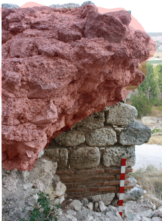
Figure 3.84 : Banded masonry of the back façade of W1.2 and the rubble heap of the later phase (red), image by author (2013).
