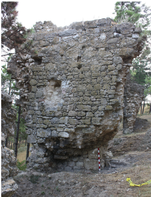
Figure 3.133 : T2.1, different masonry of the inner façade, image by author (2011).
