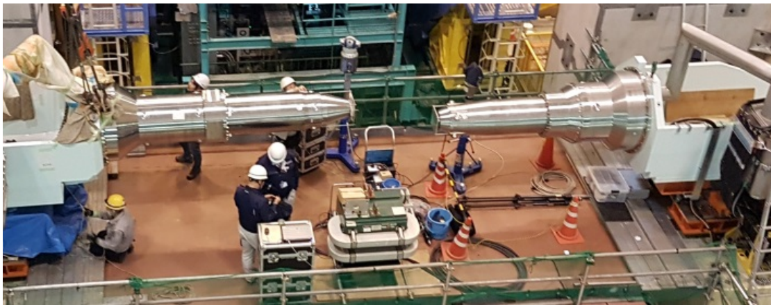
Figure 3.16: Picture of the superconducting quadrupole magnet system at the installation (February 2017) [125].
