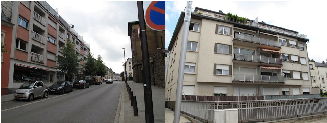
Abb. 24: Reihenhäuser in Bonnevoie
