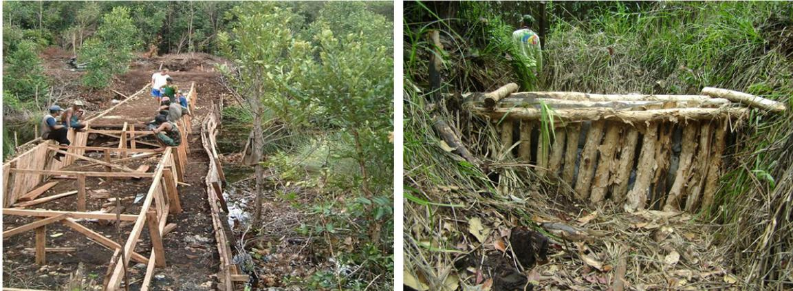
**Fig. 4** Left: Large dam constructed in a canal in the Mega Rice Project area (© Wageningen UR). Right: Example of a small dam in an illegal logging canal in the Sebangau peatland, Central Kalimantan, using locally available materials (© WWF Indonesia - Sebangau Project).
