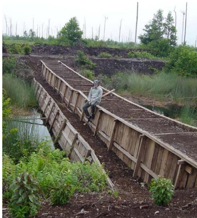
**Fig. 2** Large dam constructed across a drainage canal in degraded peatland in Block C, Mega Rice Project area. A timber frame was sealed with plastic sheeting and then filled with peat (© Kusin).
