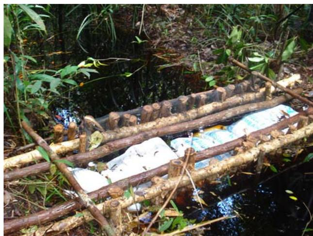
**Fig. 9** Simple dam in the Bangah catchment made of locally available material (3 m long, 1 m wide and 2.5 m deep).
