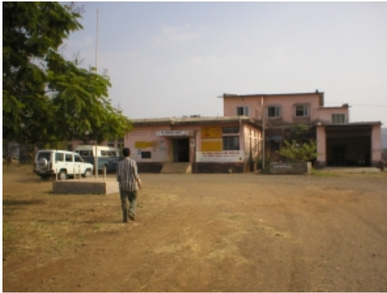
Picture 4.10: Rural Hospital Mahad, Raigarh District
