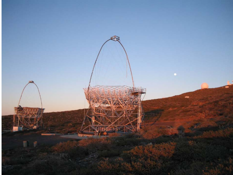
Figure 2.13: Status of the installation of the second MAGIC telescope on La Palma in spring 2006: The structure of the MAGIC II telescope seen in the foreground has been installed in December 2005, without mirrors and camera. The MAGIC-I telescope seen in the background has been taking data since 2003.
