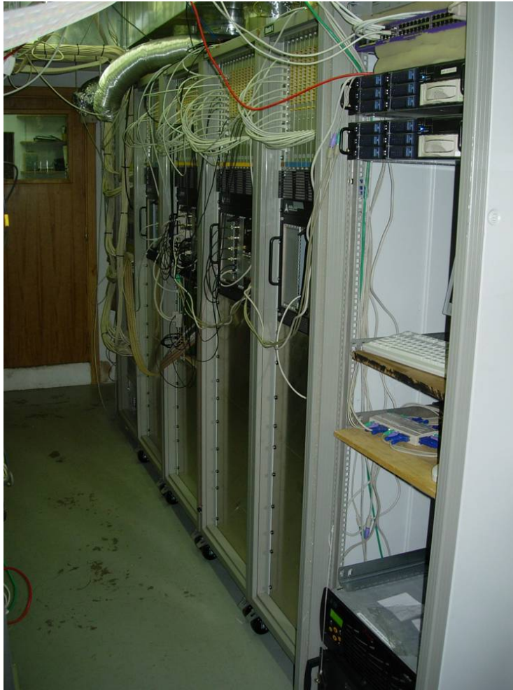
Figure 5.27: Full MUX-FADC system after installation in the electronics room of the MAGIC counting house in La Palma.
