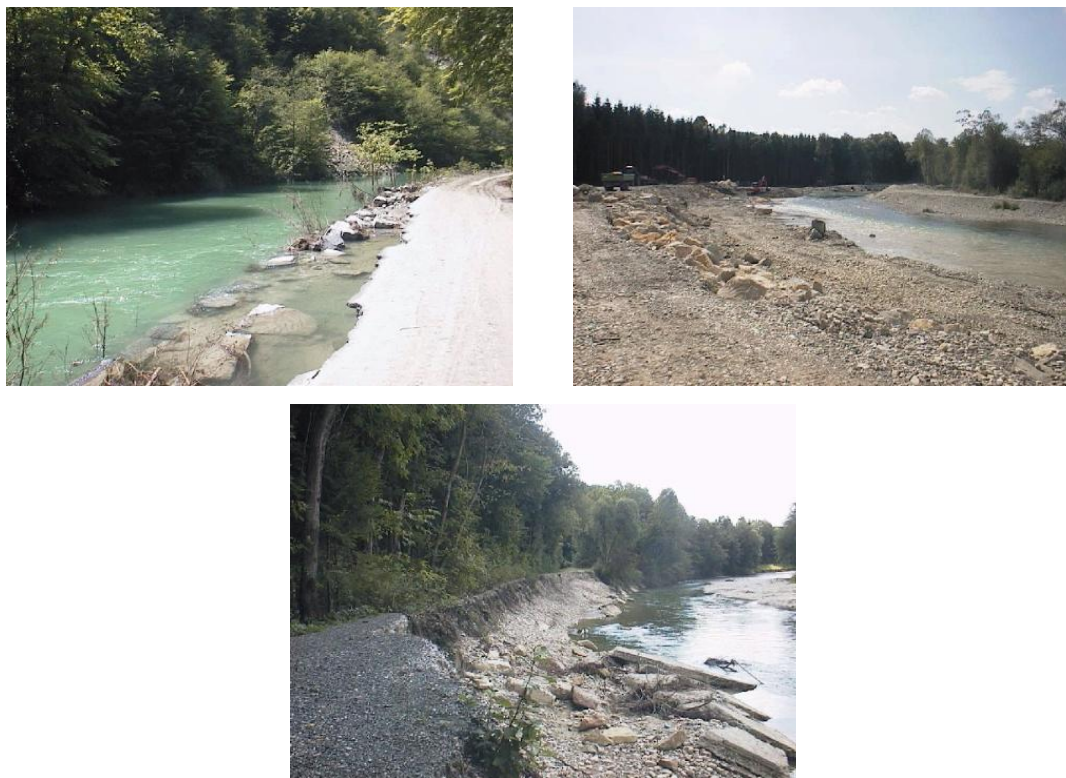
Fig. 4.5: Pictures of damages caused by the Whitsun flood in the Ammer catchment
