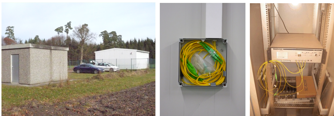
Figure 4.8: Left: View of the most southern repeater station near Münchsmünster 86 km north of Garching. Center: Fiber outlet with E2000 connectors. Right: Remotely controllable optical amplifier right before installation.
