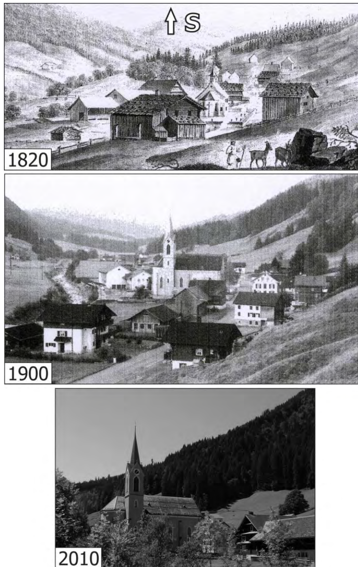
Fig. 6.2-6 Historical record of Alpthal village in the central Alp Valley (location in Fig. 3.1B). Line of sight is indicated on top of the figure. We observed an increase in forest cover especially between 1820 and 1900, and the growth of the village. 1820: Chapel of Alpthal, painting by M. Kälin (1792-1834). 1900: Photograph of Alpthal village taken from a brochure of the local authority from October 1993. 2010: Photograph in Alpthal village by R. Baran.
