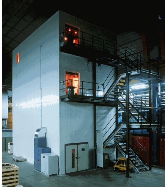
Figure 2.3: Three-Storey building of CRESST experiment
