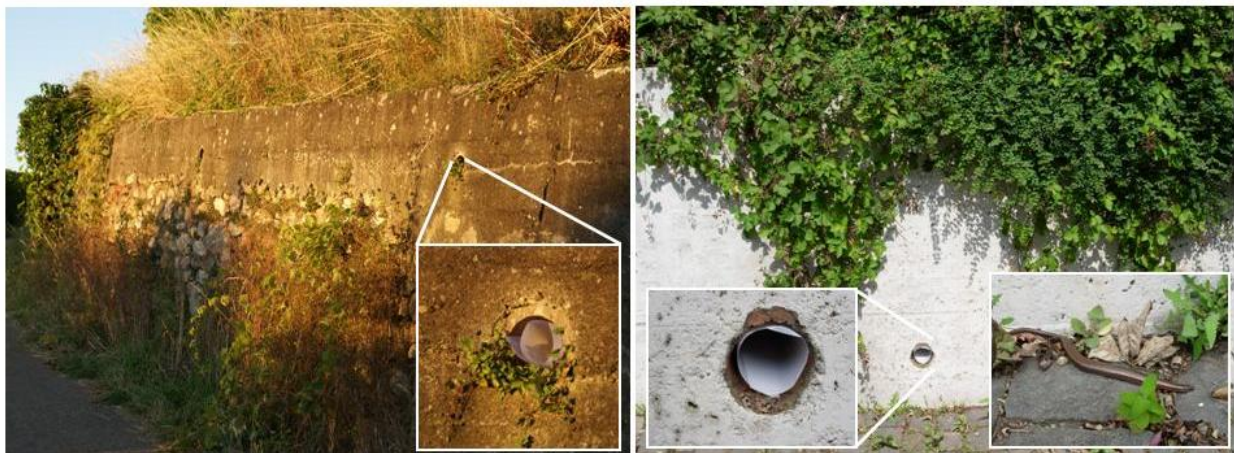
Fig. 16: Sampling site (left) stone wall with pipes, (right) concrete wall with pipe holes.
